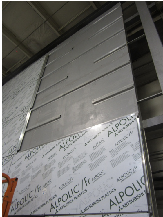
Photo No. 11 Hat Channel Spacing and Panel Installation
