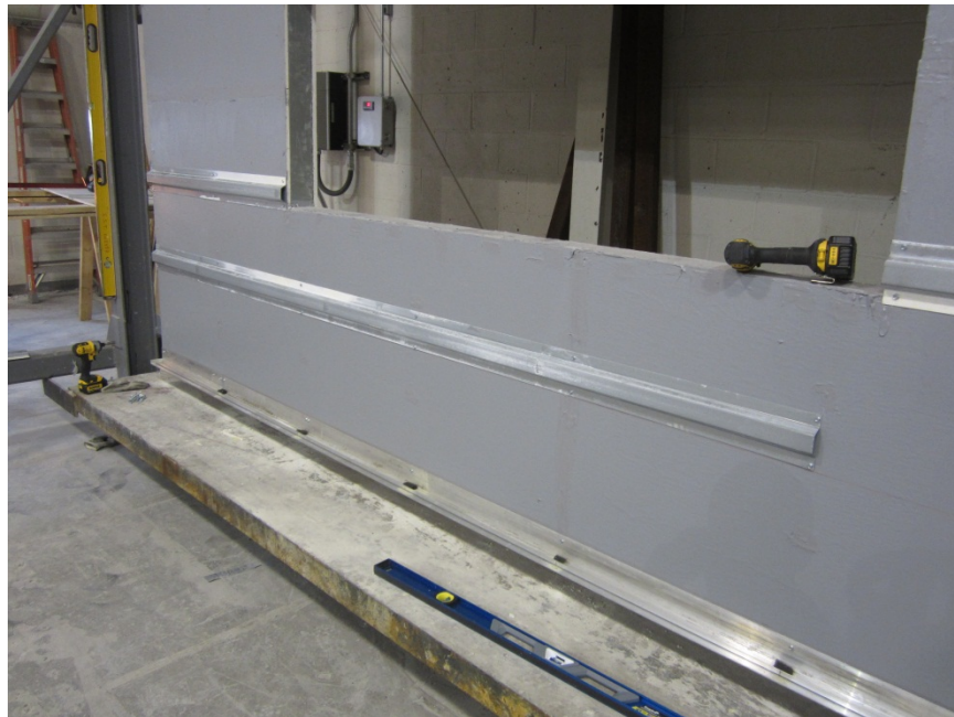
Photo No. 8 Installation of Hat Channels
