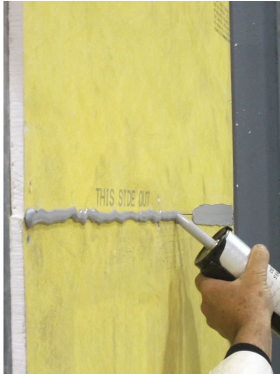
Photo No. 3 Application of Joint Sealant
