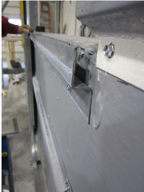
Photo No. 9 Installation of Termination Extrusion at Window Opening Sill
