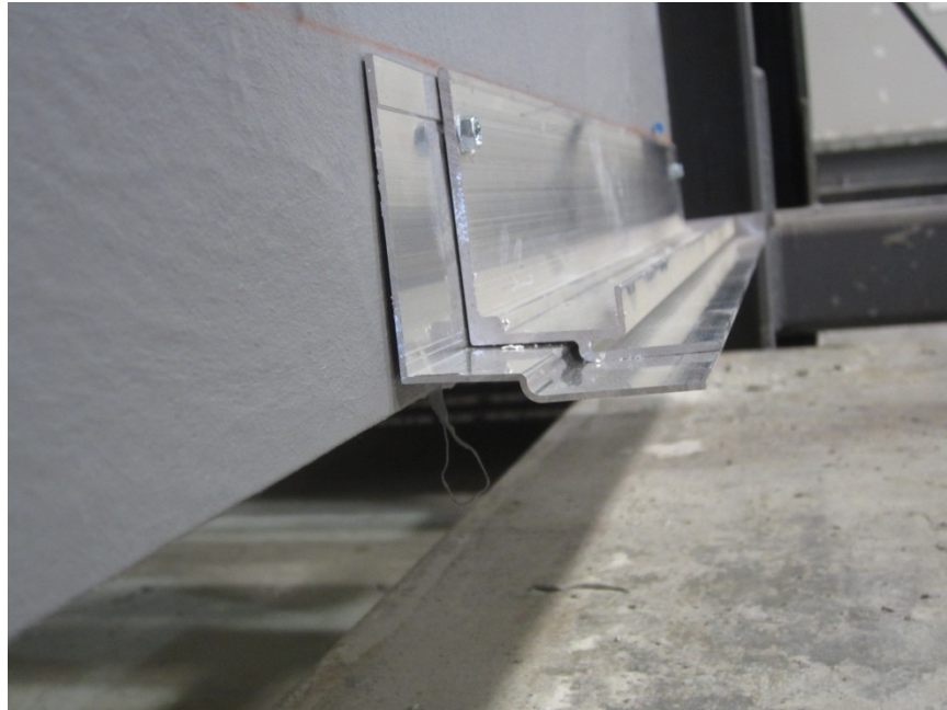
Photo No. 7 Installation of Assembly Sill Trim
