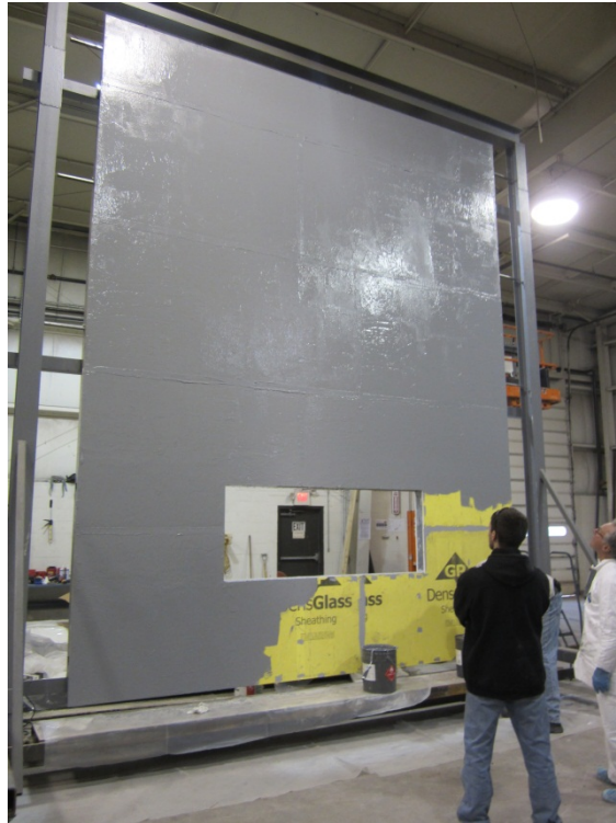
Photo No. 5 Application of Air/Vapor Barrier
