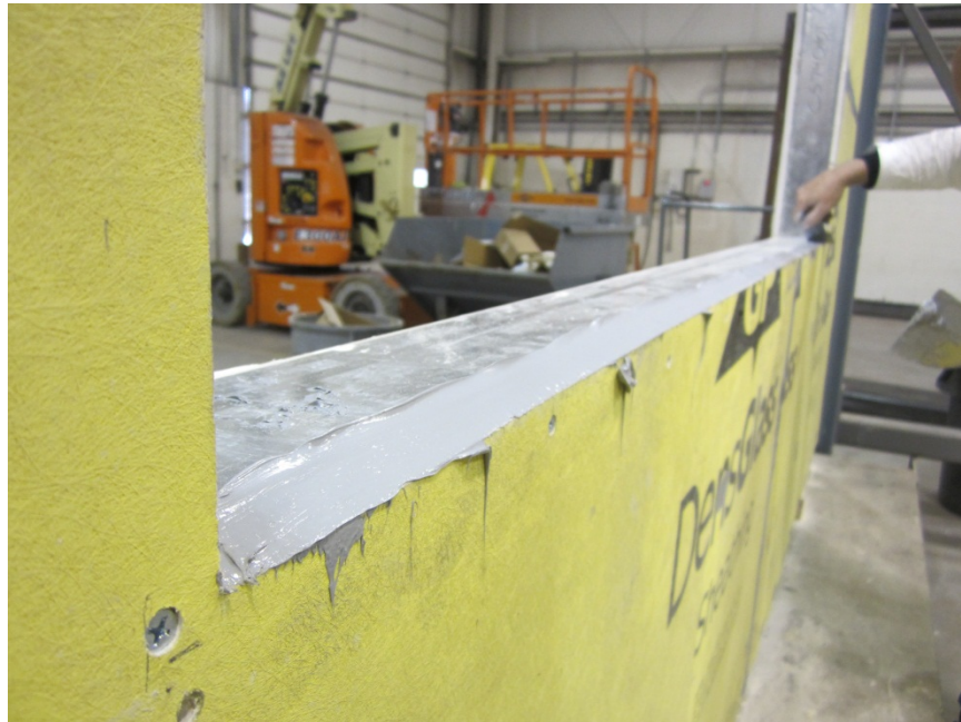
Photo No. 4 Application of Window Opening Detail Sealant
