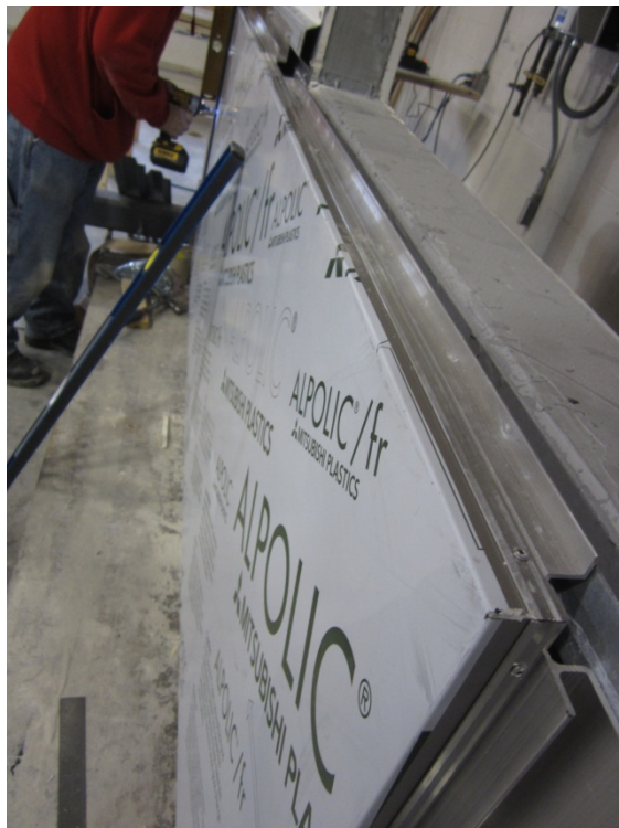
Photo No. 10 Installation of Alpolic/fr Panels www.archtest.com
