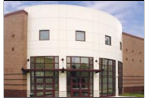
Project: Lacey Township School Architect: DiCara Rubino Architects General Contractor: Keating Builders
