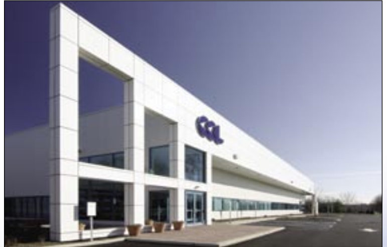
Project: CCL Label Company Architect: O'Conner / Gordon General Contractor: Worthington Construction
