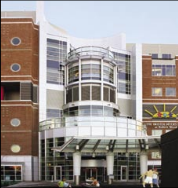
Project: RWJ Children's Hospital Architect: Granary Associates Architects General Contractor: Wm Blanchard Company
