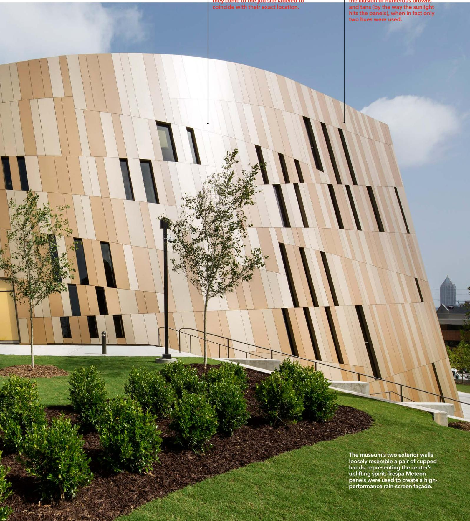
The museum's two exterior walls loosely resemble a pair of cupped hands, representing the center's uplifting spirit. Trespa Meteon panels were used to create a high-performance rain-screen façade.
