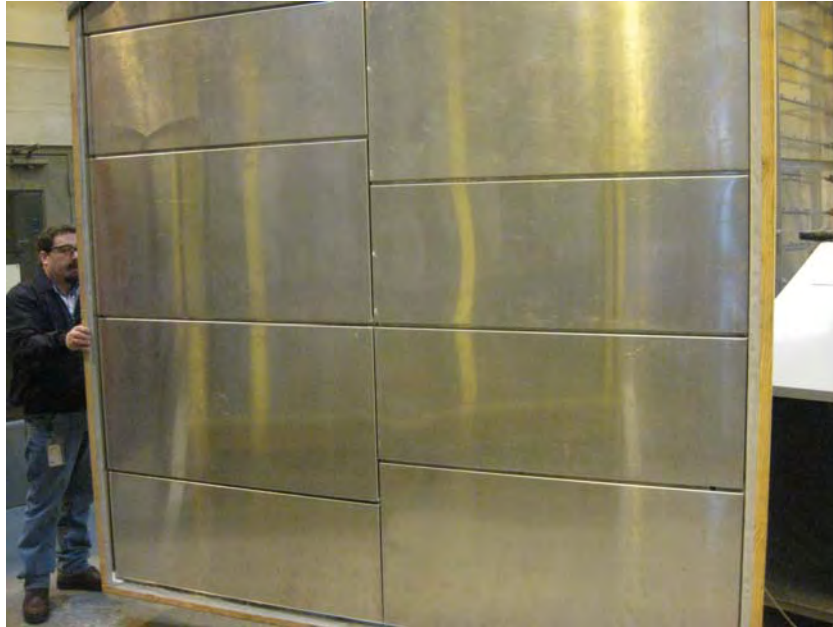
Photo No. 1 Exterior View of Tested Wall System
