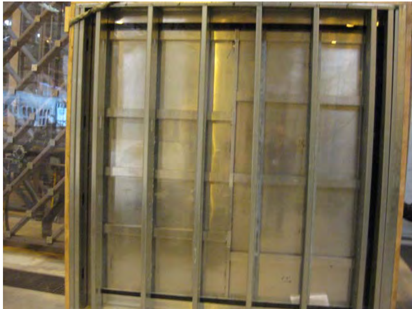
Photo No. 2 Interior View of Tested Wall System
