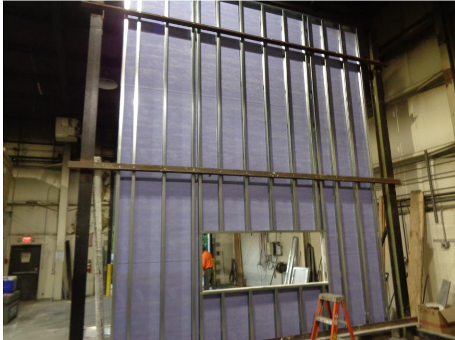
Photo No. 1 Core Wall Construction
