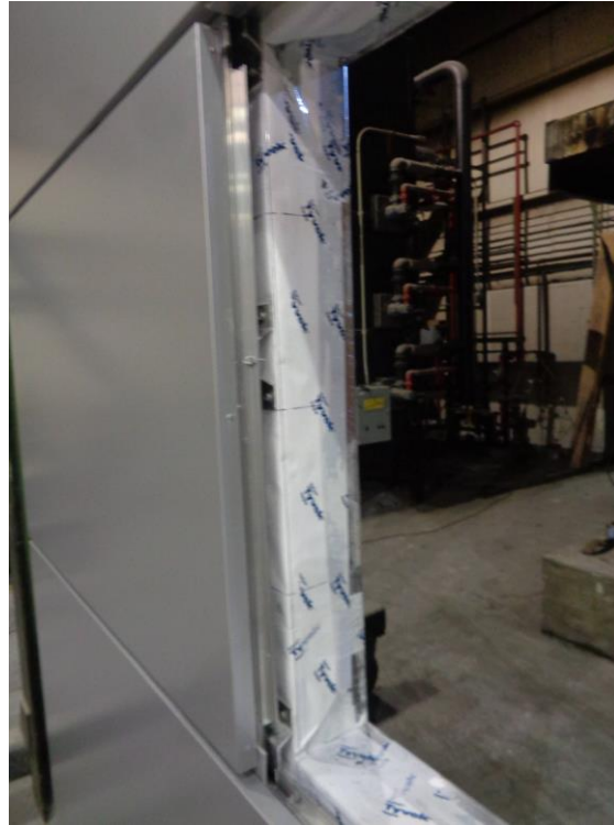
Photo No. 5 Panel Installation at the Window Opening
