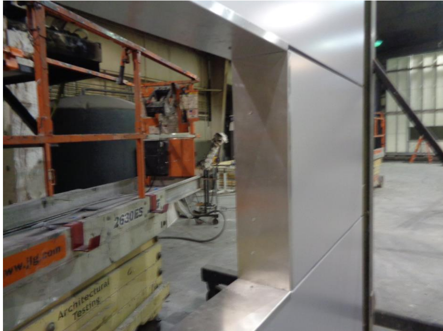
Photo No. 7 Window Opening Flashing
