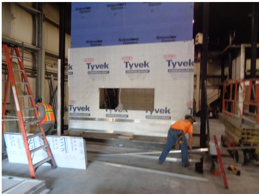
Photo No. 2 Installation of Dupont™ Tyvek® CommercialWrap®
