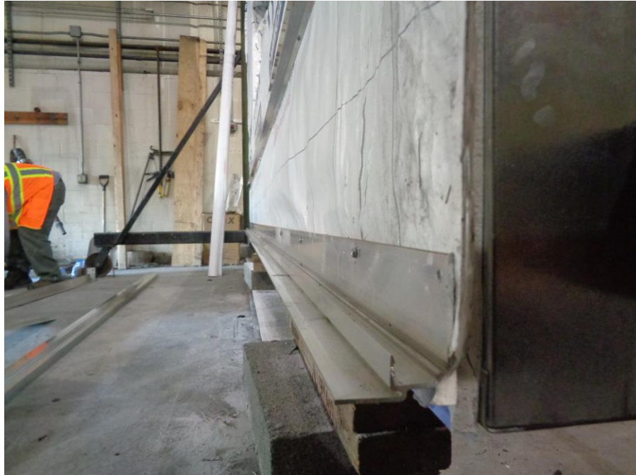
Photo No. 3 Installation of Bamco DX-5400 Extrusion
