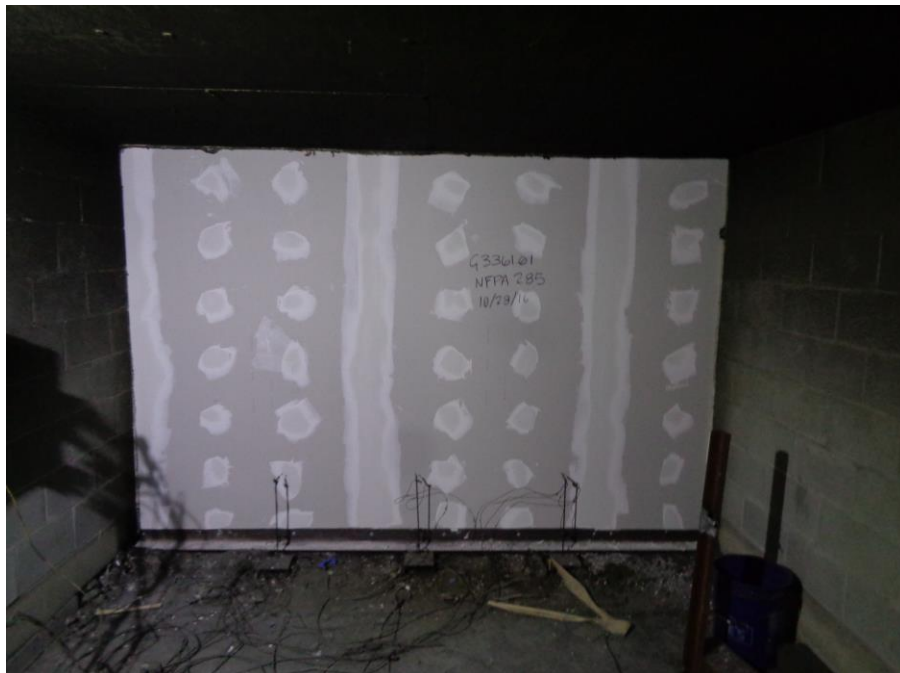
Photo No. 10 Interior Second Story (Pre-test)
